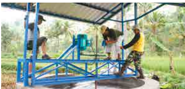
YTLJT staff monitoring a micro hydro unit
