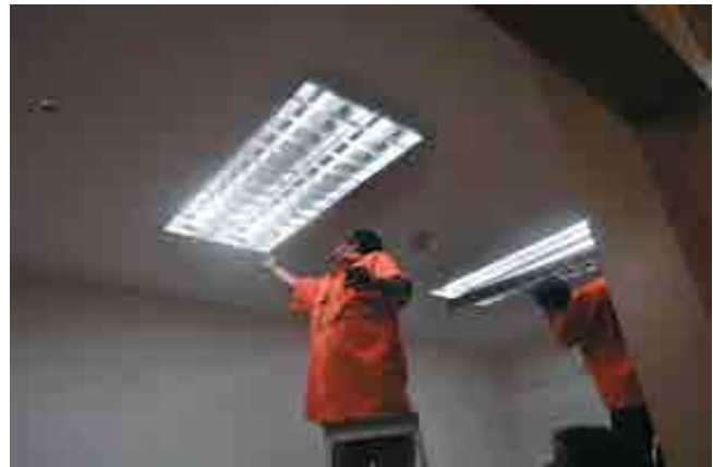
The installation of high-efficiency lights at one of the six customers' offices
