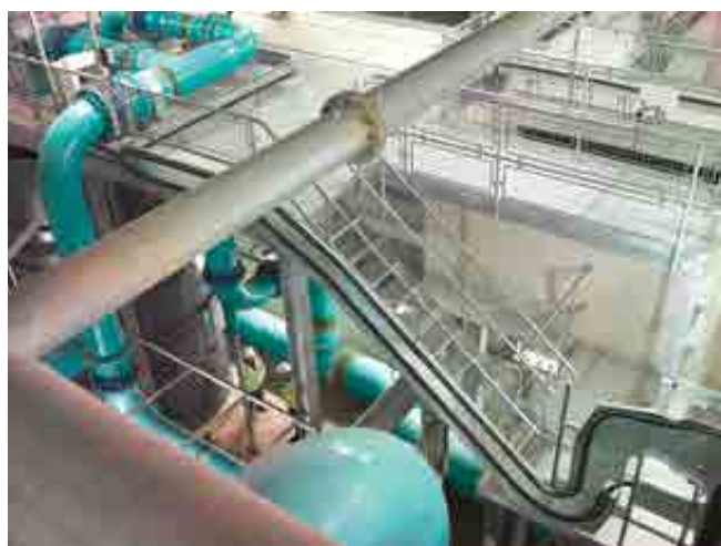
Wessex Water's energy team inspecting the Maundown water treatment works which supplies clean water to nearly 200,000 people across Somerset
