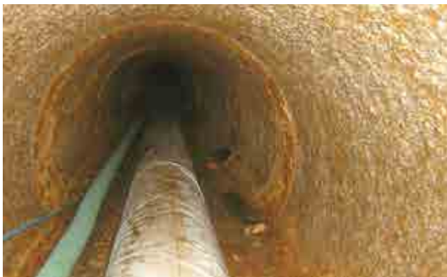
Wessex Water's infrastructure – Inflated UV liner within a structural pre-liner as it passes along the floor of the culvert
