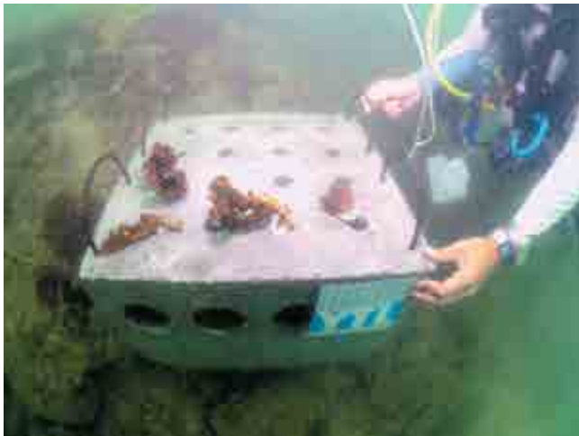
The specially designed and fabricated green cement blocks weighing approximately 20 kg each, cast, transported and delivered by YTL Cement and placed in the sea with nubbins attached
