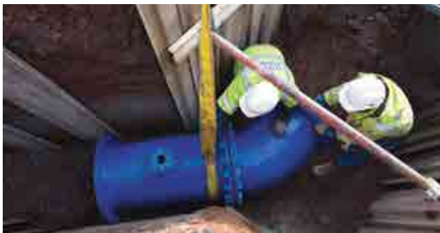
Wessex Water staff installing new water mains
