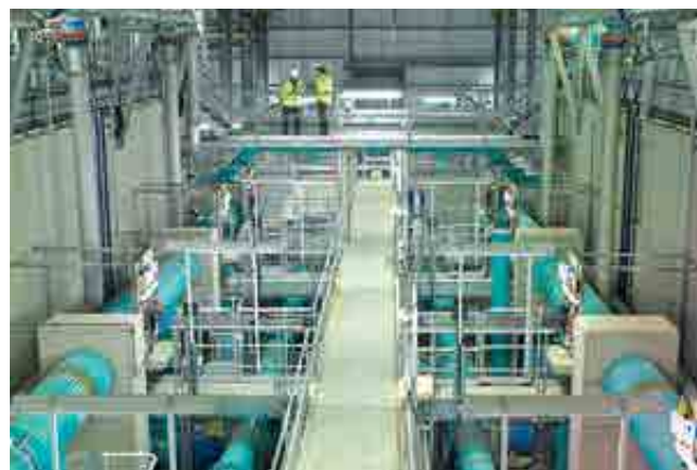
Wessex Water staff consistently monitor the plants energy usage
