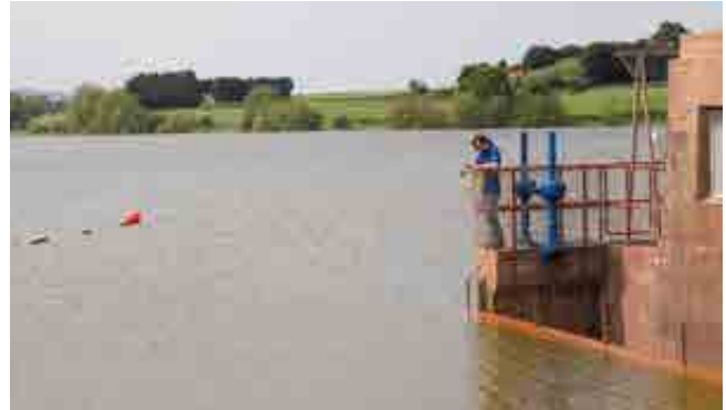
Wessex Water staff monitoring the water quality at Durleigh reservoir
