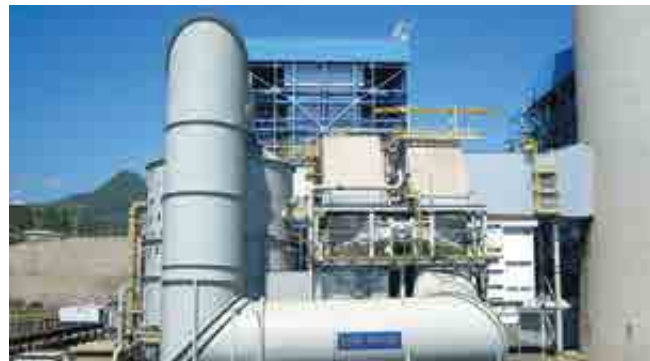
PT Jawa Paiton II Power Station, the first power plant in Indonesia certified with ISO 50001
