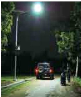
Solar cell street lamps at Klompangan Bhinor
